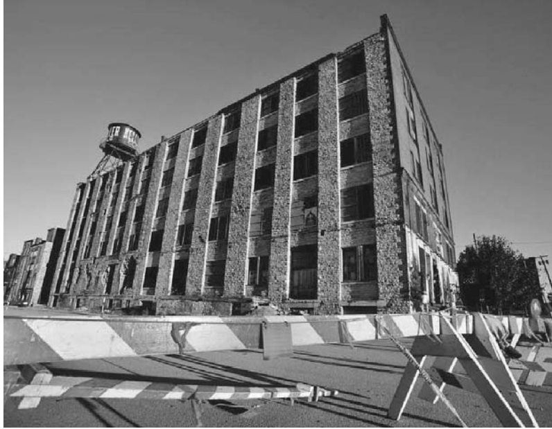
The old Keller Building.
